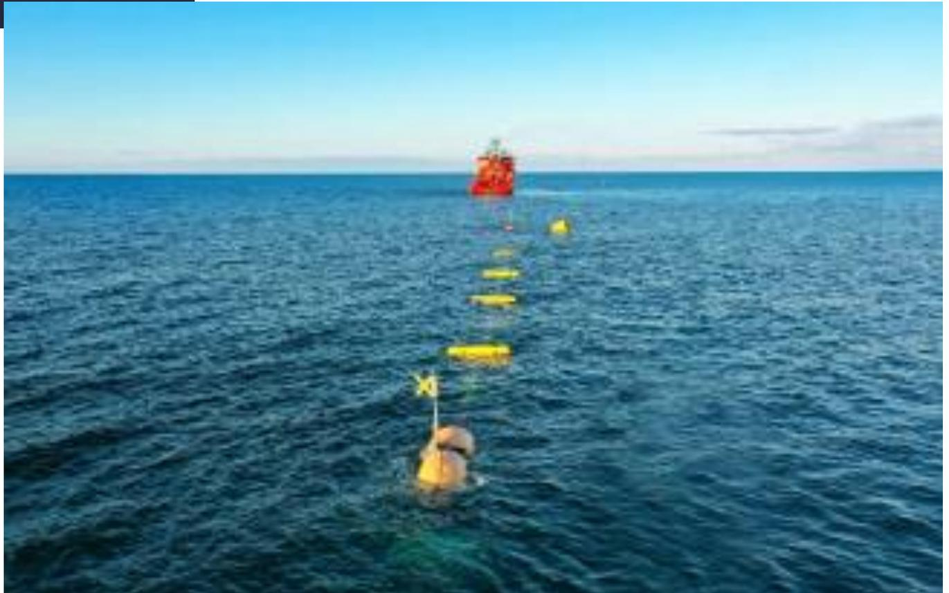
Deployment of the first H24 wave energy converter
